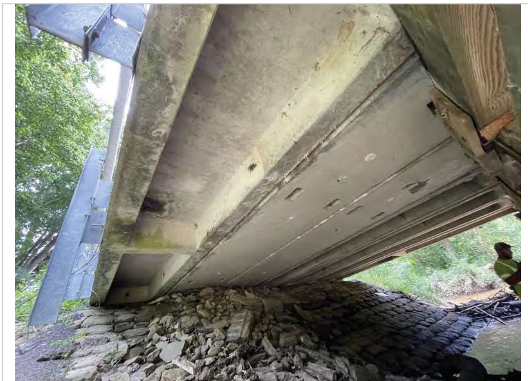
Bottom deck span #4
