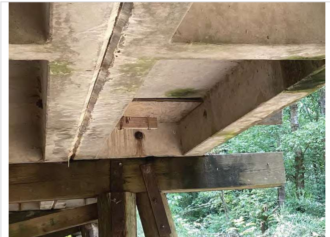
Span 2 slab G patched area
