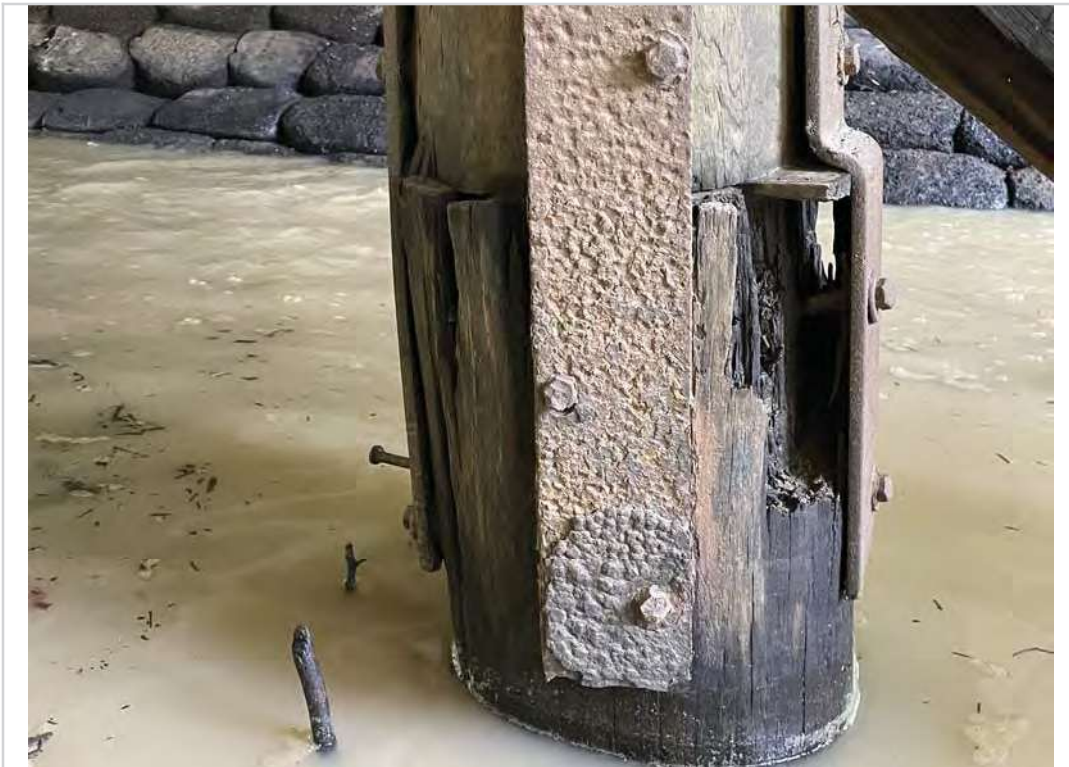
Bent #3 pile "D"
