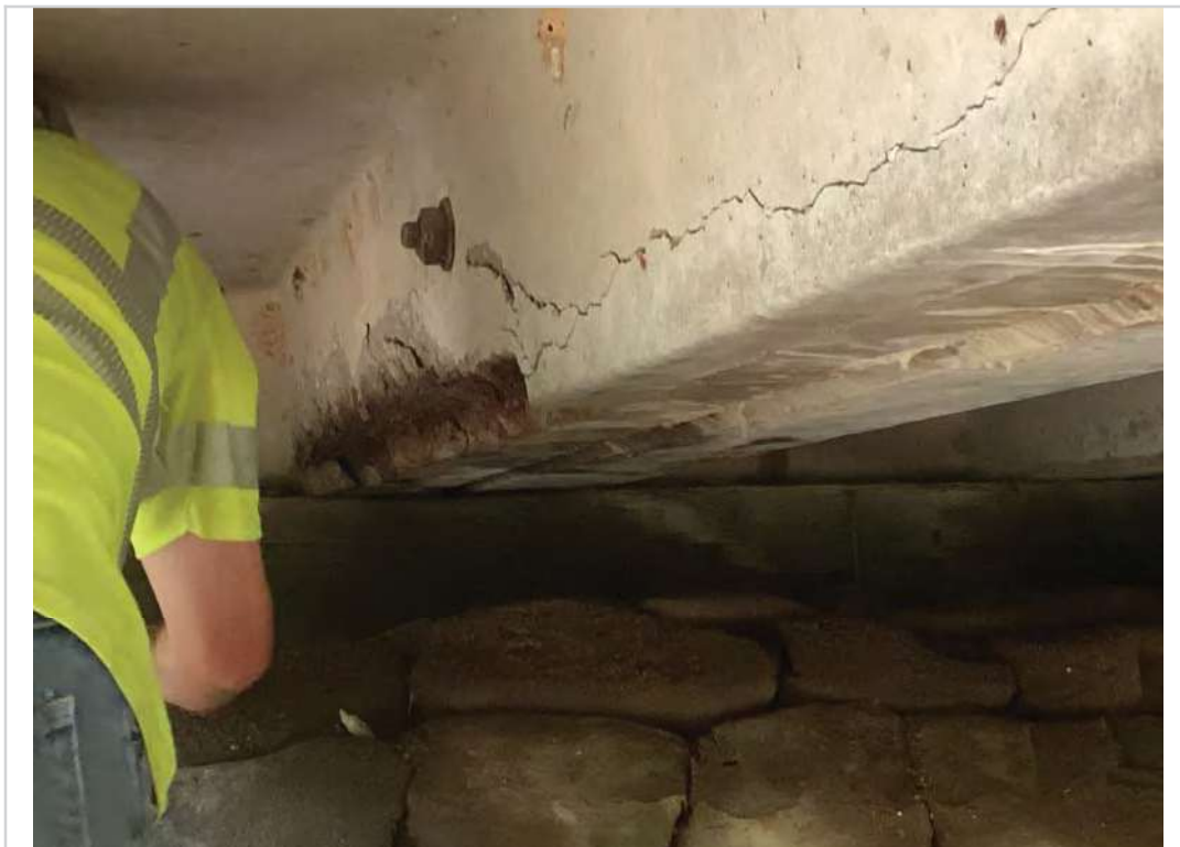
Span 1 slab G spall to steel
